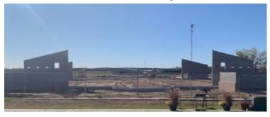
**Photo** of the north side of the worship space **rising up** from the foundation. The concrete is involved in the exterior walls of the worship space and the gathering space and utility and HVAC space on the north side of the worship space.
